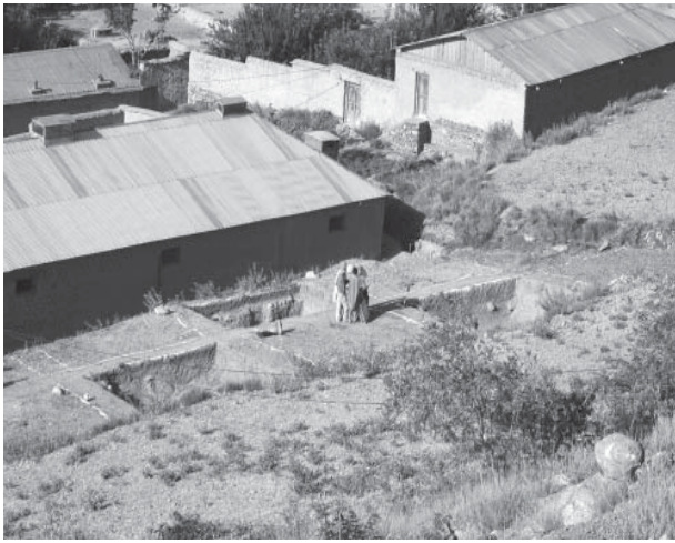
General view of GTC site
