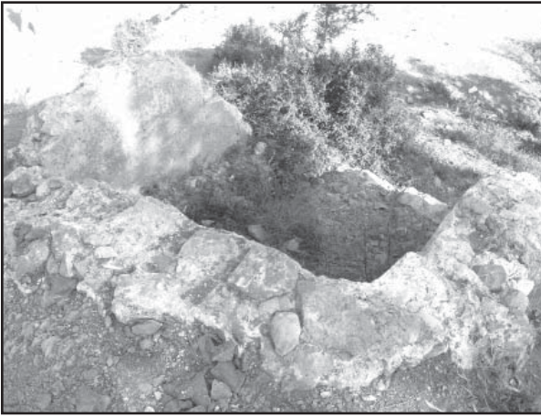
31. Chhajjian Water Tank (# 156)
