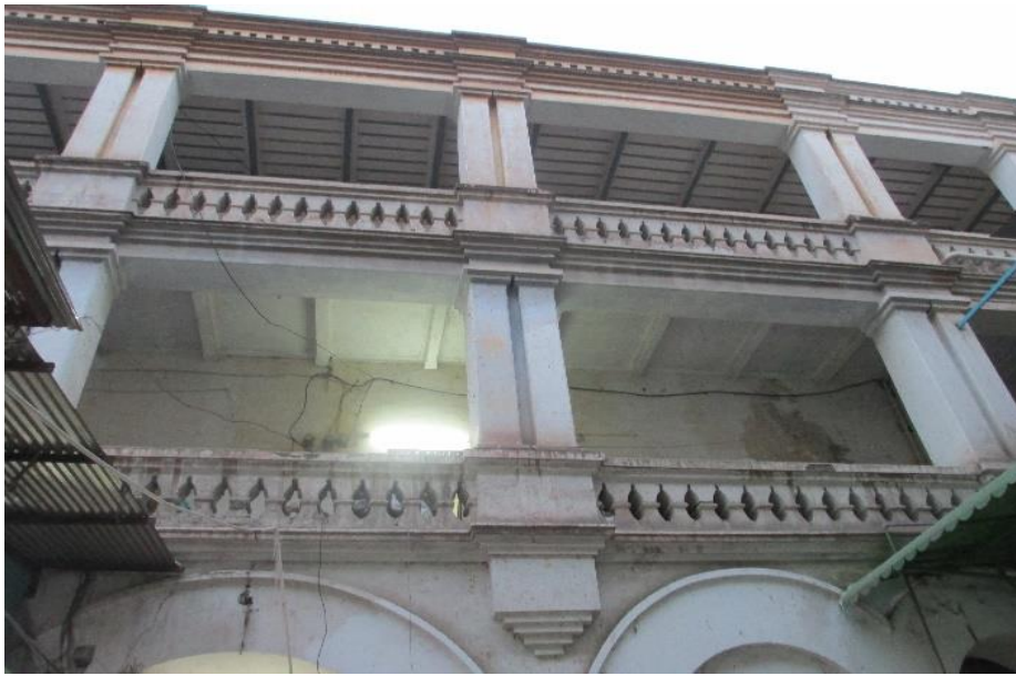
Figure 7: Interior view, showing multi stories of the Building
