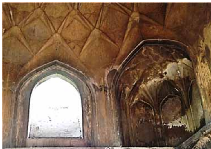
Figure 11: Squinches below the dome
