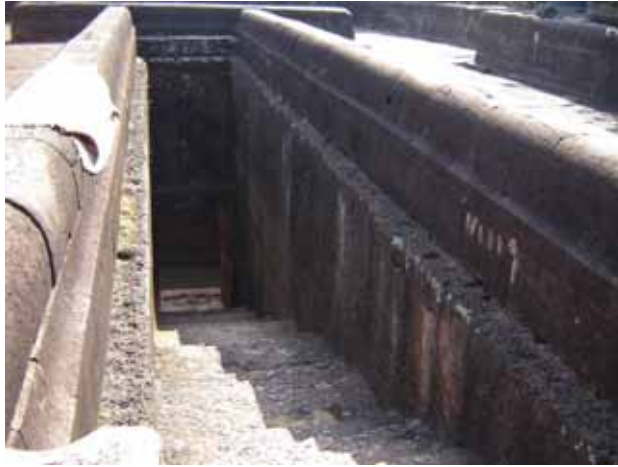
Plate 3. Stepwell at Udaygiri (Photograph by author)
