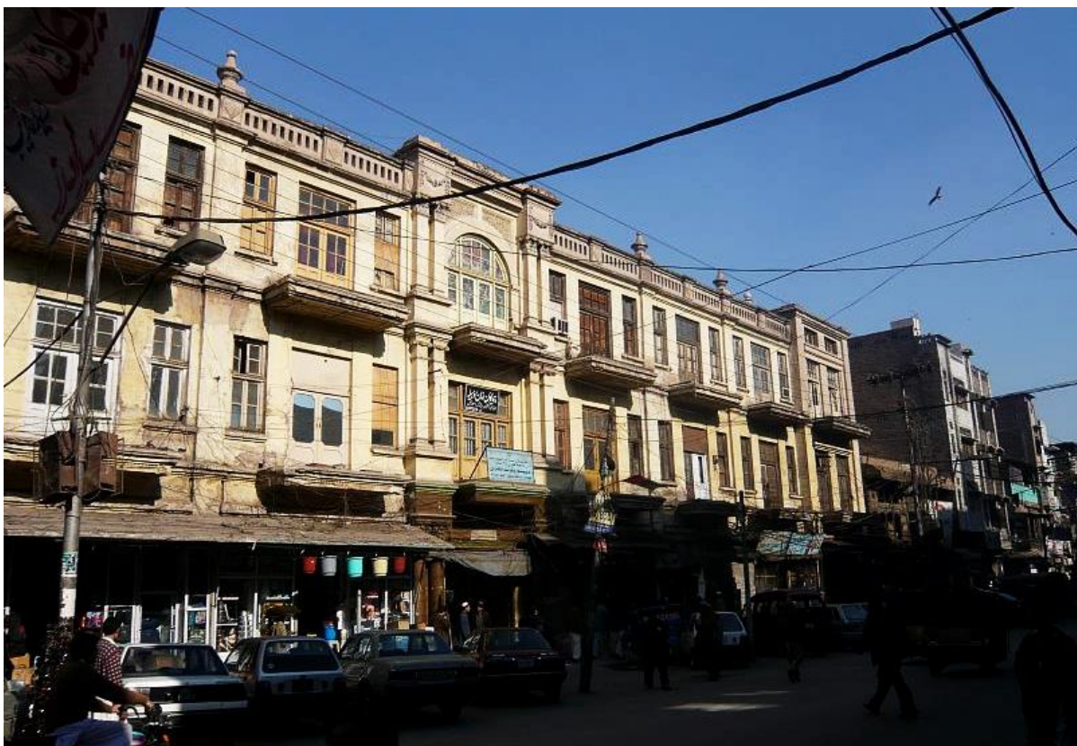
Figure 4: Façade of the Building.
