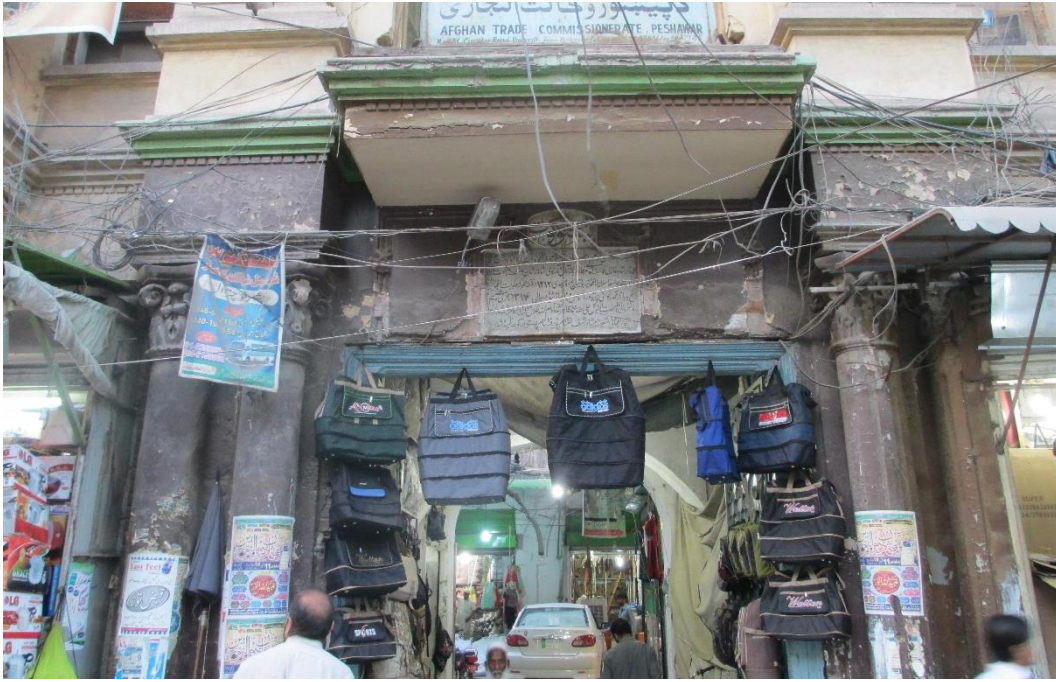
Figure 5: Main entrance showing white marble slab inscription with Corinthian pilasters on either side.
