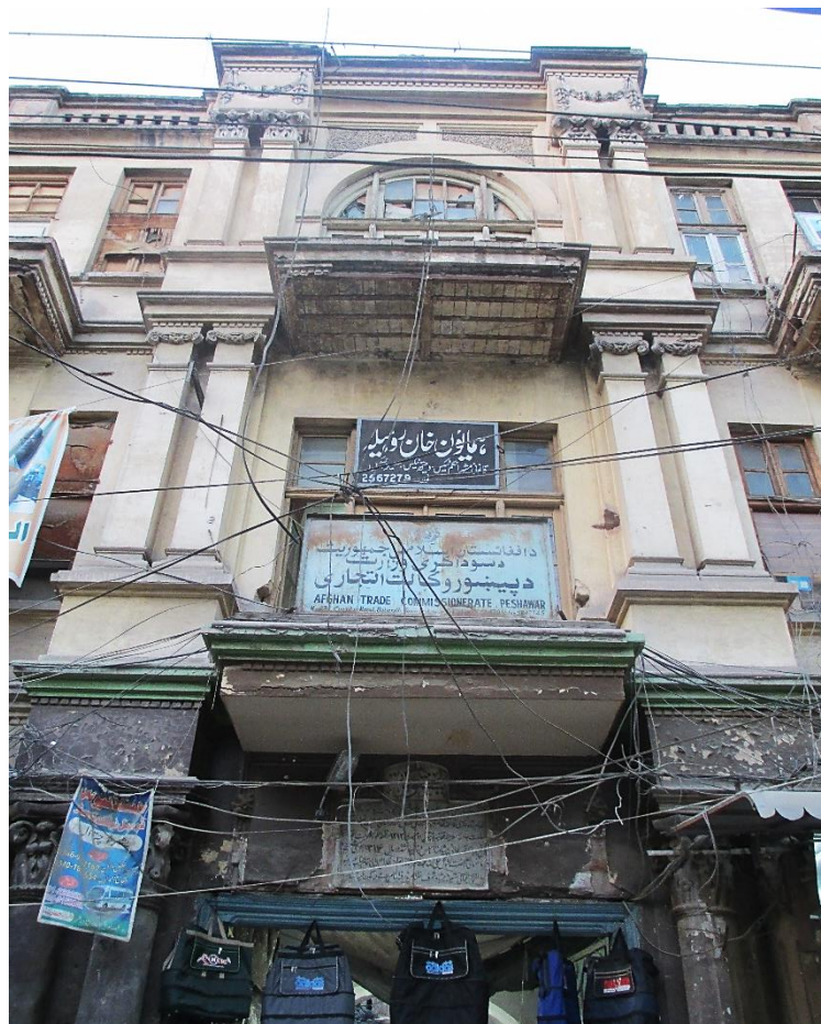
Figure 6: Complete view of the main entrance with rest of the storey
