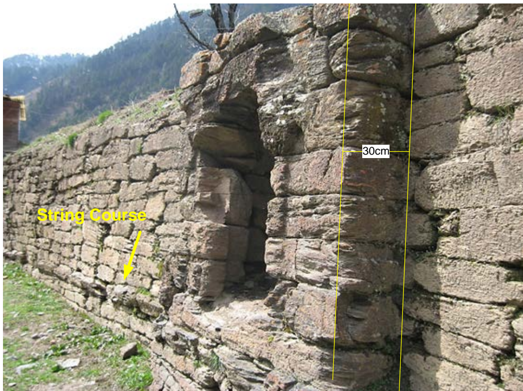
Figure 8. Northern wall and the niche
