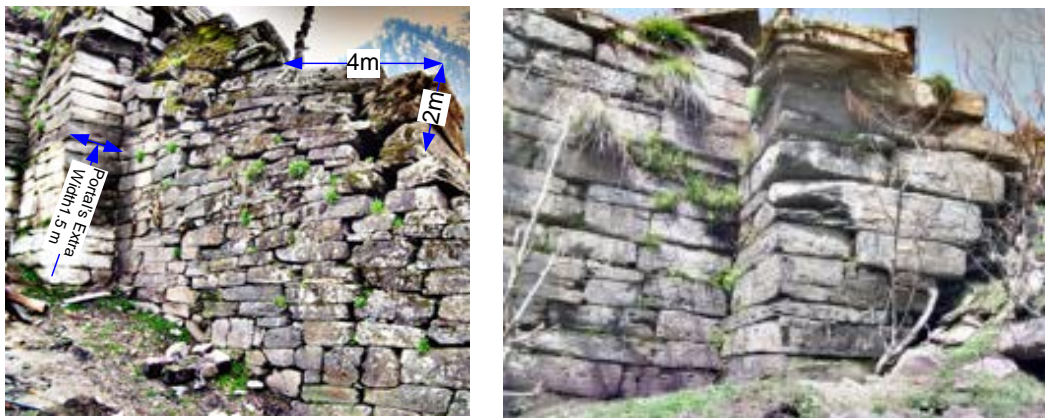
Figure 2: Staircase joining the portal's podium. A view of northern and southern faces respectively.
