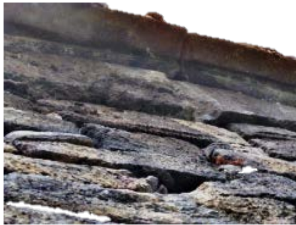
Figure 7. Coping in the Northern Wall
