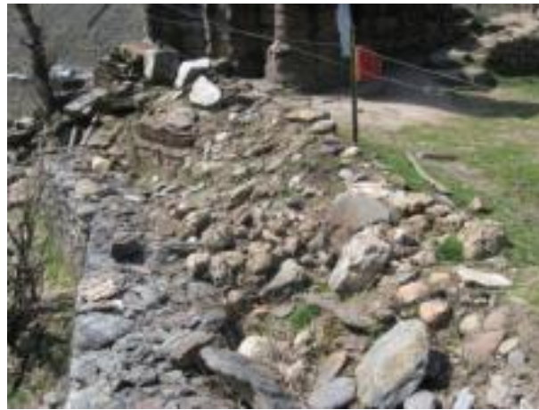
Figure 10. Reinforcements for southern wall
