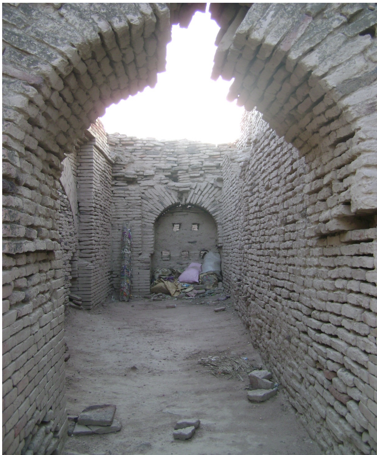
Figure 5. Barrel vault Of the Tomb of Khalid b. Walid. Kabir Wala, Punjab,
